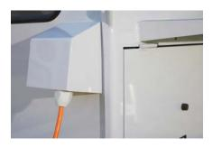
A 16A three-phase electrical connection provides power to all the equipment in the cabin.
